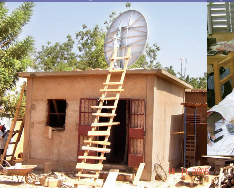
Left: installation of the VSAT in Ouahigouya
